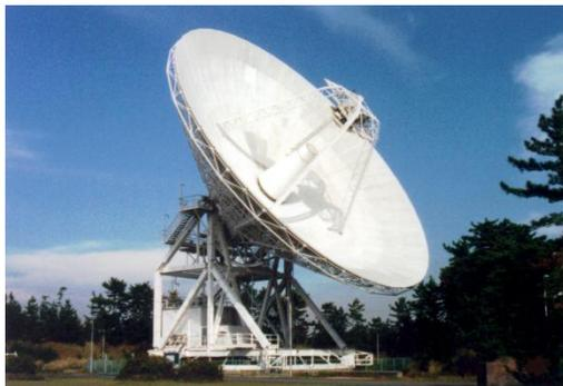
**Figure 2-1: 34 m. aperture antenna in Kashima Space Research Center**
