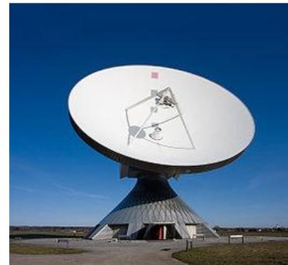
Figure 2-10: High-gain reflector antenna used for radio, television and data communications
